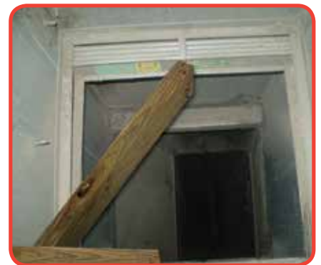
Fire Dampers Inspection
